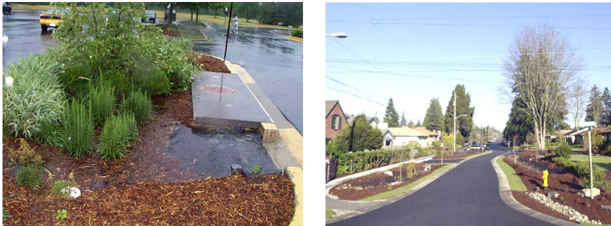
Figure 1. Working Bioretention cells in an urban, left, and residential, right, application. (Source: Michael Clar, P.E, Ecosite, Inc., Ellicott City, Maryland)
